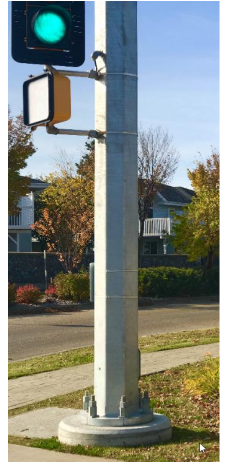
Traffic lights installed
