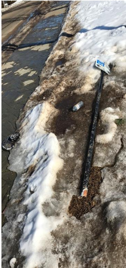
Traffic signs fixed
